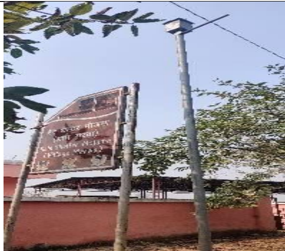
Picture A.2: Stolen Solar Panel of a Solar Street Light near Rain Shelter, Mojma, Bihar
