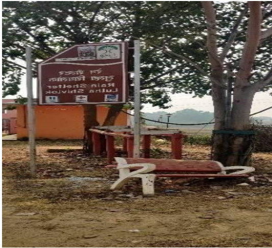
Picture A.1: Broken RCC Bench nearby Rain Shelter, Lulha Shivlok, Bihar
